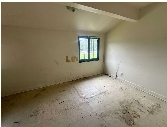
11. EXAMPLE OF MOISTURE DAMAGED FLOORING
