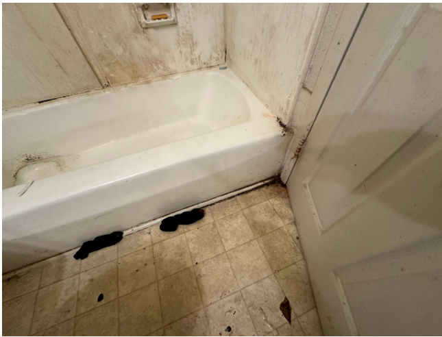
25. EXAMPLE OF MOISTURE DAMAGED FLOORING
