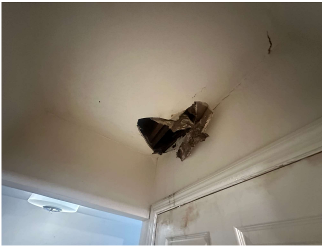
13. EXAMPLE OF MOISTURE DAMAGED CEILING
