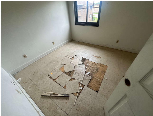
27. EXAMPLE OF MOISTURE DAMAGED FLOORING
