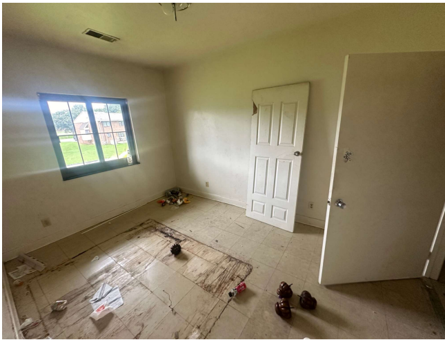
31. EXAMPLE OF MOISTURE DAMAGE FLOORING
