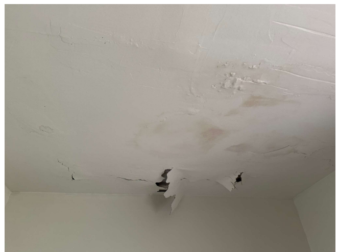
18. EXAMPLE OF SUSPECT ORGANIC GROWTH AND MOISTURE DAMAGED CEILING
