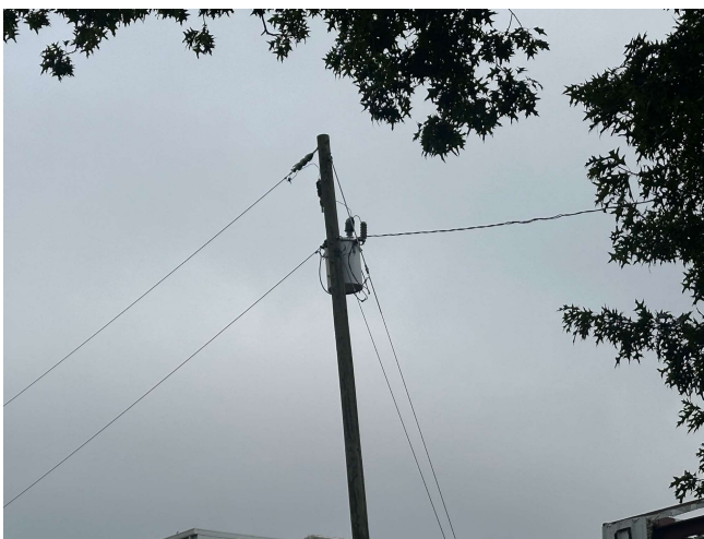
47. TYPICAL POLE MOUNTED TRANSFORMER
