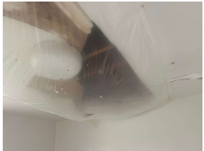
16. EXAMPLE OF MOISTURE DAMAGED CEILING
