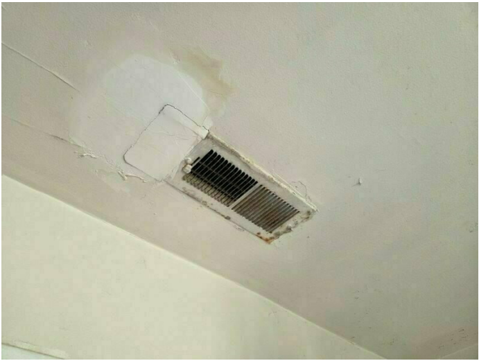
34. Typical multi-family interior with microbial growth
